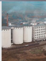
One of COWI's first groundbreaking projects was the Ostenfeld Silo. Despite its huge dimensions, the walls were just 25 centimetres thick, making it significantly cheaper to build. Using prestressed concrete, the walls could bear the pressure from within and remain sealed. A choice of material which later turned out to be useful for more than just silos.
