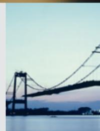
In 1960, two suspension bridges at Uttamo and Pargas in Finland marked a breakthrough for the firm's bridge division, shaping the design of the first of two iconic bridges in Denmark; the Little Belt Bridge. The pylon legs rise 121 metres above sea level. At 70,000 tonnes each, the two buried anchor blocks resist 17,000 tonnes of force from the main cables.
