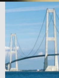
Tying the eastern and western part of Denmark together, the 18 kilometre Great Belt Link, with a main span of 1,624 metres, was designed to have the world's longest suspension span at the time of construction. Taking tricky aerodynamics into account, designing for large ship impact, operating road and rail, and protecting the marine environment, the Great Belt Link became a reality, breaking new ground for bridge engineering.
