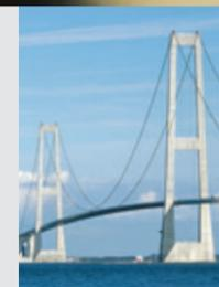
Tying the eastern and western part of Denmark together, the 18 kilometre Great Belt Link, with a main span of 1,624 metres, was designed to have the world's longest suspension span at the time of construction. Taking tricky aerodynamics into account, designing for large ship impact, operating road and rail, and protecting the marine environment, the Great Belt Link became a reality, breaking new ground for bridge engineering.
